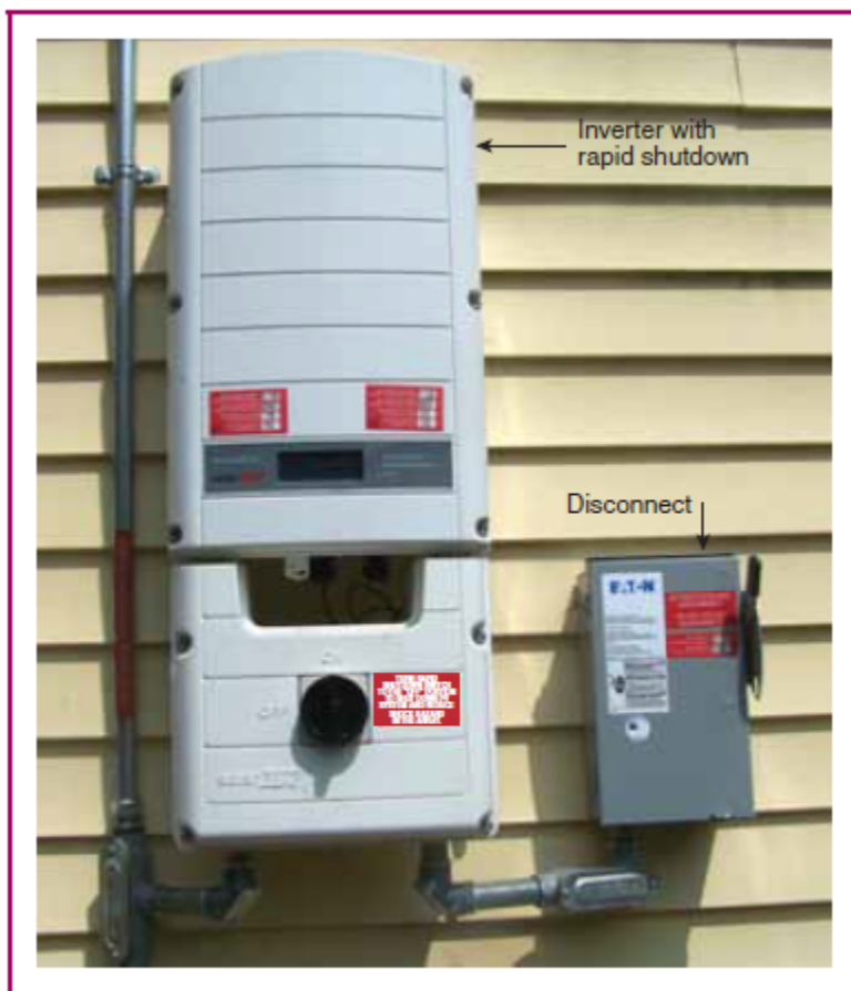
EXHIBIT 690.3 An interactive inverter. (Inverter courtesy of SolarEdge Technologies; Photo courtesy of Michael and Diane Mello)
