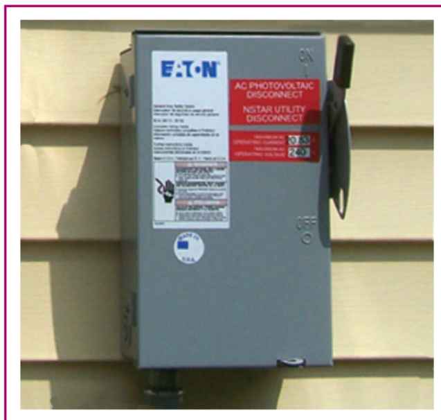
EXHIBIT 690.10 PV system disconnect.
